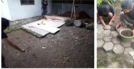
Figure 3. Site Preparation Source: Author
