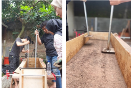
Figure 8. Formwork Dissembling After 24 Hours Source: Author
