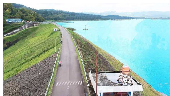
Figure 1. Wadaslintang Dam, Wonosobo, Central Java, Indonesia.
