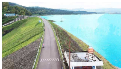
Figure 1. Wadaslintang Dam, Wonosobo, Central Java, Indonesia.
